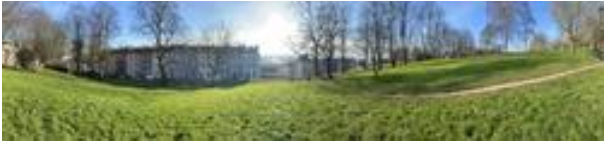
Panoramic shot from Brandon Hill showing Georgian terraces of Queens Parade and York Place and view through site to hills beyond Bristol
