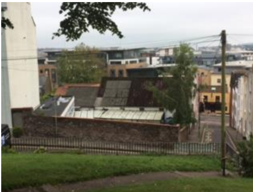
Daytime view across site
