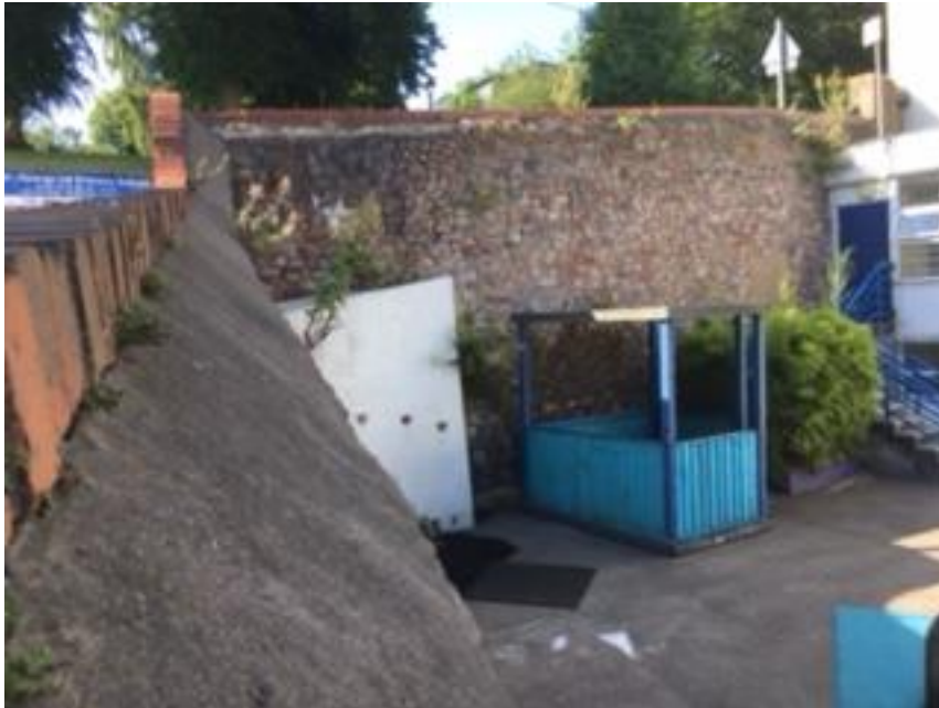
Rear of boundary/retaining wall onto Queens Parade 2021
