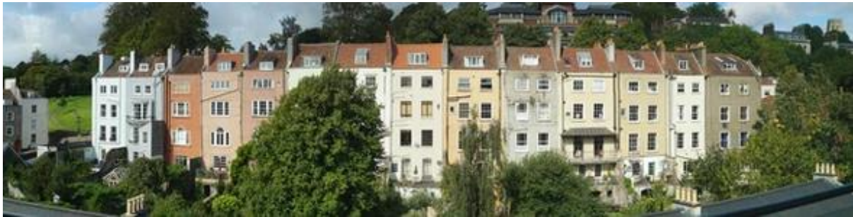
View of Queens Parade from rear with views through and over site to greenery on Brandon Hill
